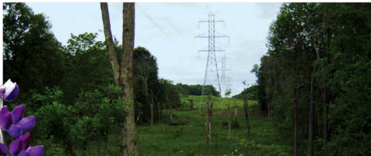
The cleared corridor.
