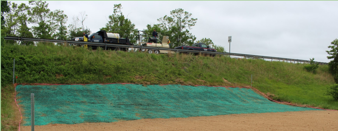
Figure 3.6 Hydroseeded slope along US Route 6.
