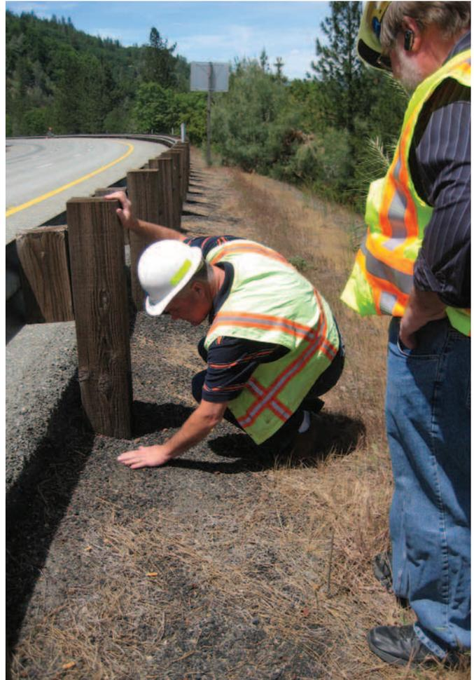
*Caltrans employees inspecting the performance of a vegetation control mat installed under an existing guardrail along highway.*
